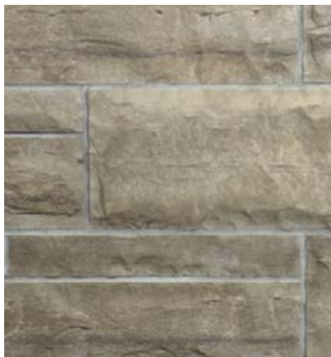
Peninsula Masonry Blend
